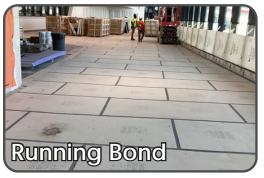
SkudoBoard 4x8 can be installed stack bond or running bond (offset). Skudo recommends leaving an expansion gap of 1/16th "as boards can expand in extremely hot conditions.
