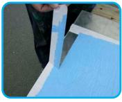
4. Remove the masking tape while the product is still wet. This helps to achieve a good thick edge that is easier to peel when the product is no longer required.
