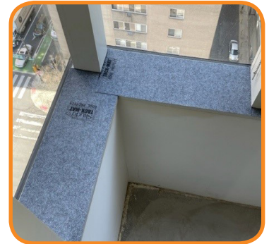
Protect edges from damage
