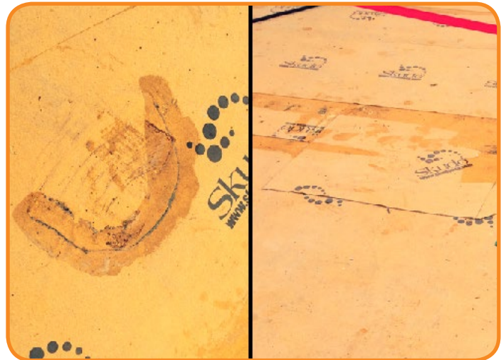
Inspect daily for tears and patch/repair if needed
