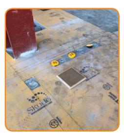
Adheres and remains stationary • Use for all types of construction layouts • Fire Retardant No need to worry about staining • Won't rub off or wash away • Antibacterial/Antimicrobial
