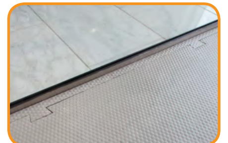
Edge pieces fill in gaps along walls
