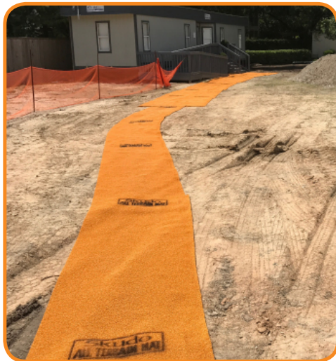
Walkways - Commercial Construction
