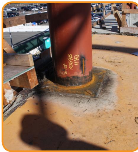
Protection Against Welding
