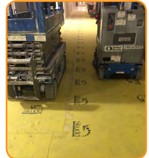
Under Light Machinery
