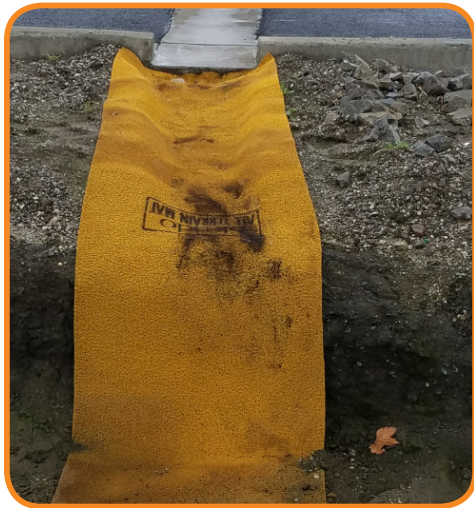
Water Run-Off Areas
