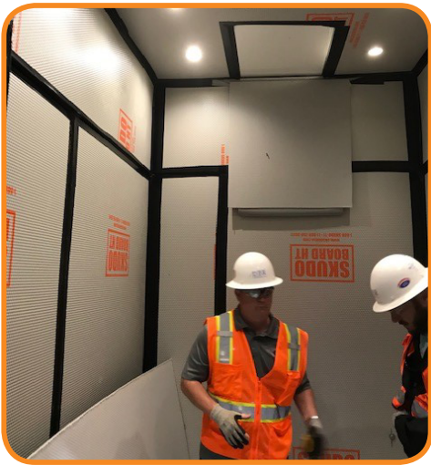
Vertical Protection (Freight Elevator)
