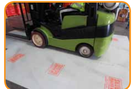
Superior protection under forklift and construction traffic
