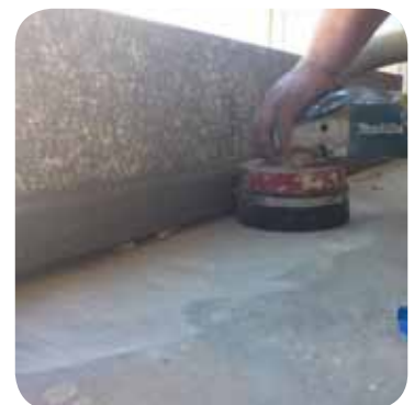
Protect edges from damage
