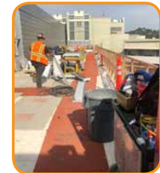
Safely Direct Traffic through a Jobsite - including TPO Roofs
