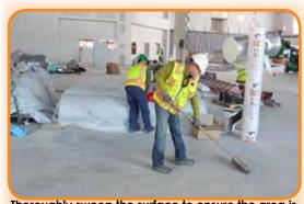
Thoroughly sweep the surface to ensure the area is clean and free of debris/foreign materials that will compromise and contaminate the Base Coat.
