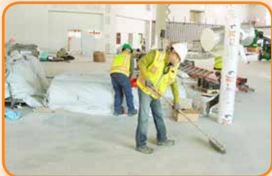
Thoroughly sweep the surface to ensure the area is clean and free of debris/foreign materials that will compromise and contaminate the Base Coat.
