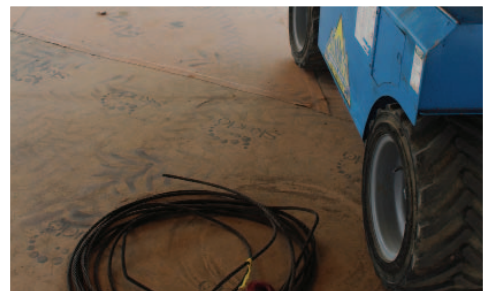
Machinery and fire marks do not damage the concrete
