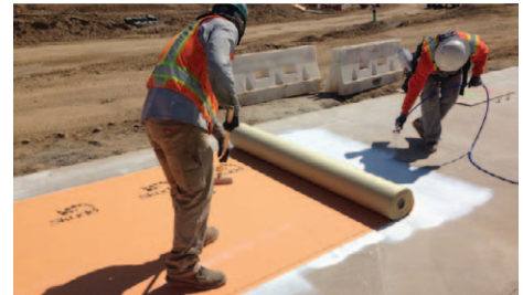
Applying 40,000 s.f. of HT Commercial System
