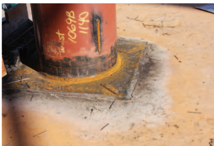
The HT Mat protected the surface from welding slag
