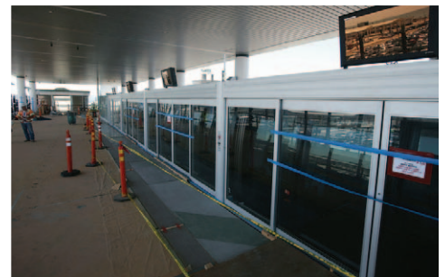
Station fit out partially complete
