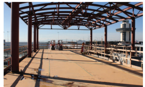
Skudo ready for work to begin at the Oakland station
