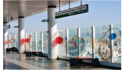
Finished polished concrete & tile on the Oakland station
