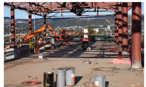
Skudo holding up to construction at the Coliseum station
