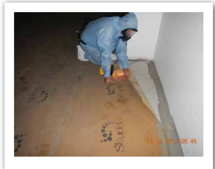
Tile protected with Skudo HT Mat is undamaged
