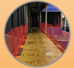
Exterior Concrete Driveways Skudo HT Commercial System SkudoBoard Standard
