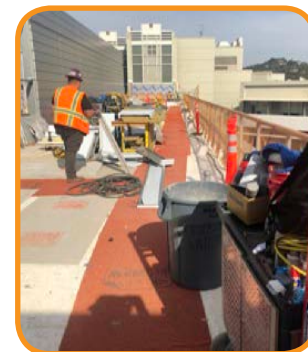
Safely Direct Traffic through a Jobsite - including TPO Roofs
