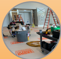
Hospital Corridor SkudoBoard Interlock
