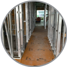
Under Walls/Framing Skudo HT Commercial System
