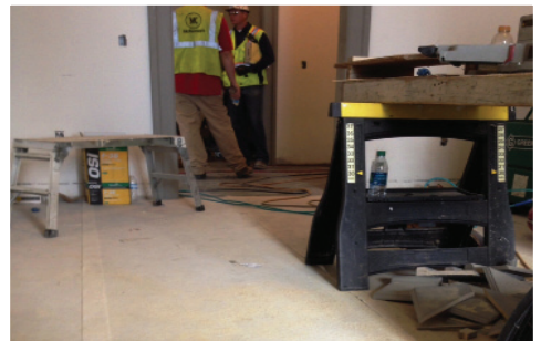
Tack-Mat provides protection against dust and dropped materials
